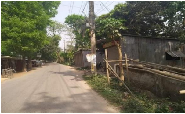
Fig. 5: No Lane Marking but Roadside Hazards (Road # 1)
