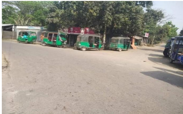
Fig. 6: No Channelization at The Intersection, No Marking (Road # 1)
