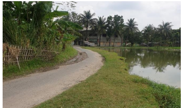
Fig. 18: Pond Along the Roadside Without Crash Barriers (Road # 8)
