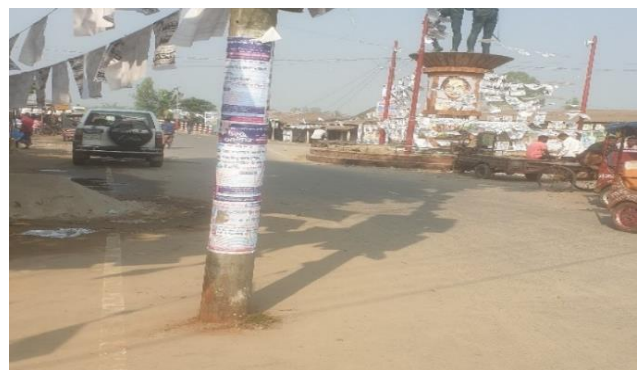
Fig. 20: Utility Pole on the Carriageway (Road # 4)
