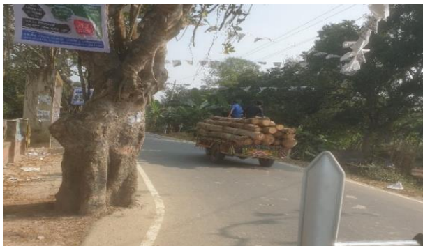
Fig. 7: Roadside Hazards, No Clear Zone (Road # 4)
