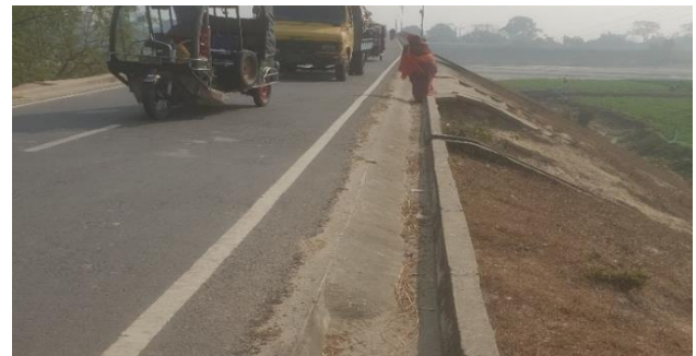
Fig. 19: Open Surface Drain, Steep Fill Slope, No Barriers (Road # 4)
