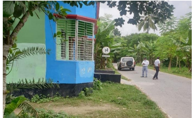
Fig 9: Lack of Pedestrian Facilities on Hilly Roads (Road # 6)
